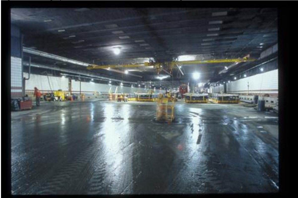
Figure 6: Photograph of the Thomas O'Neill Tunnel during construction
