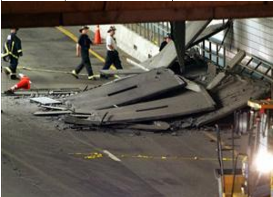
Figure 10: Workers walk from a Big Dig tunnel in Boston on 11 July 2006. Cement ceiling panels fell from the open area visible in the center of the photo
