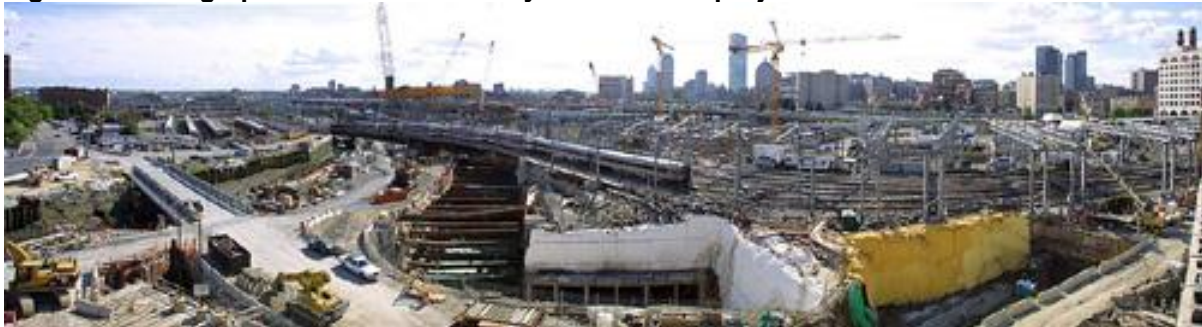
Figure 8: Photograph of the Central Artery construction project
