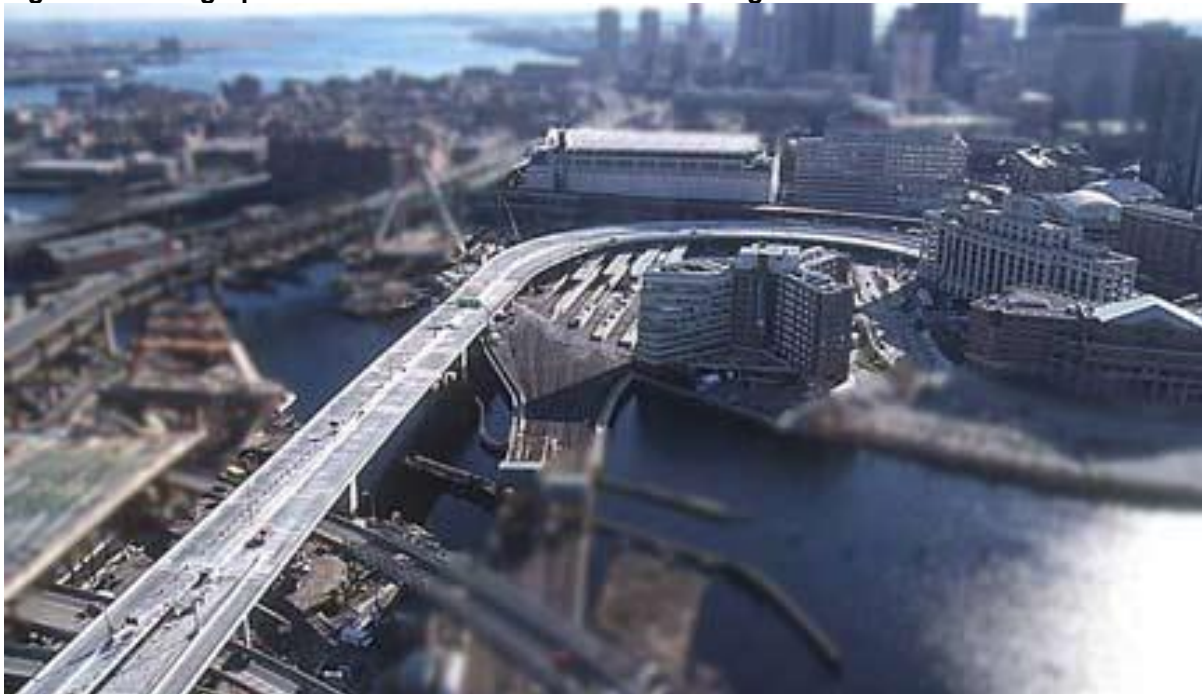
Figure 4: Photograph of the Leverett Circle Connector Bridge
