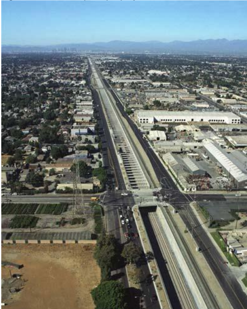
Figure 2: View of the principal project infrastructure - trench
