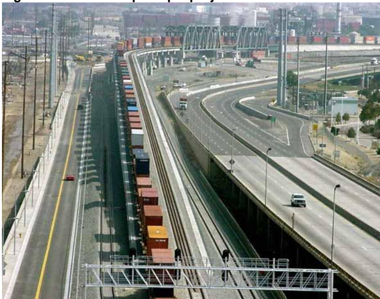
Figure 1: View of the principal project infrastructure – rails
