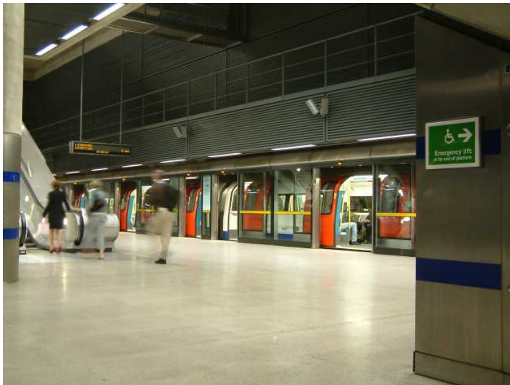
Figure 40: Platform with Safety Barriers at Canary Wharf Station
