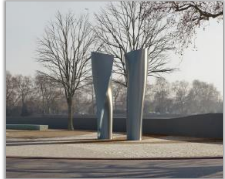
Signature ventilation columns
