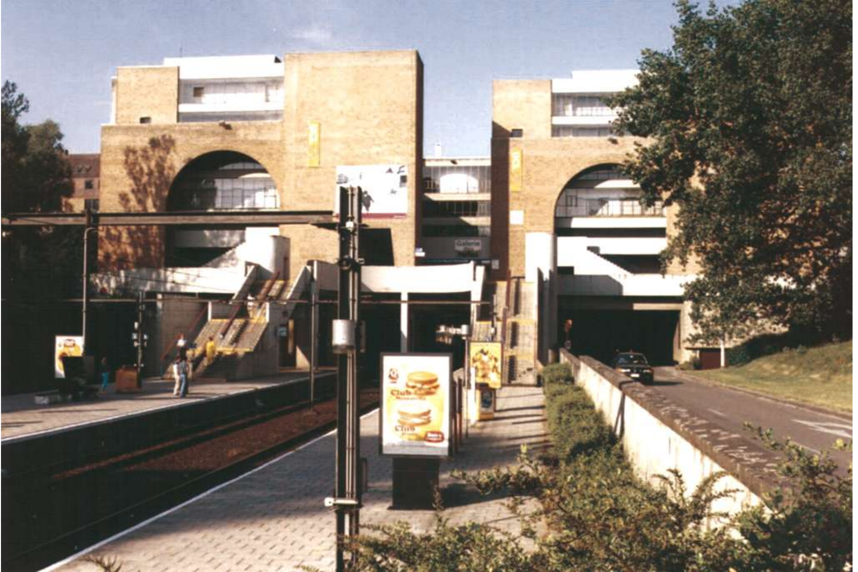
The new station (1976). It is entirely underground, in view of being covered at a later stage.
