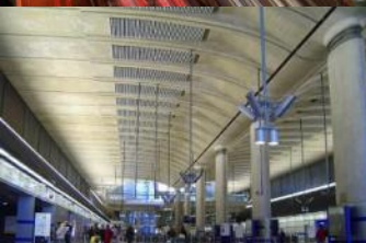
Jubilee Line Extension (UK)
