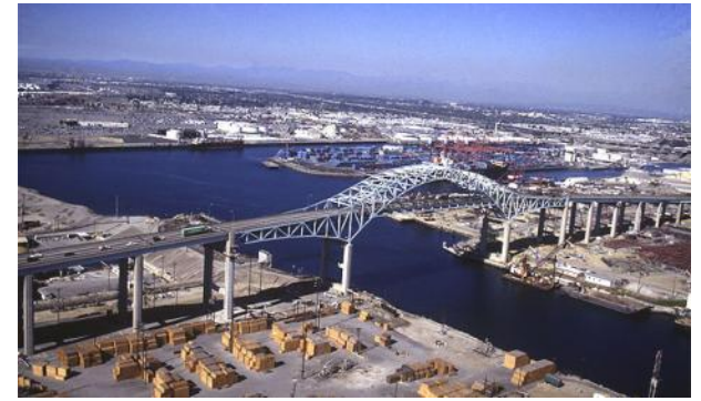
Alameda Rail Corridor (USA)
