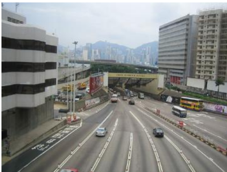
Western Harbour Tunnel (HK)
