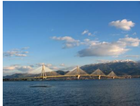
Rion Antirrhion Bridge (GR)
