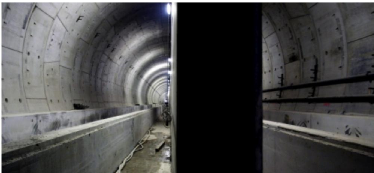
Figure 8: inside the tunnel
