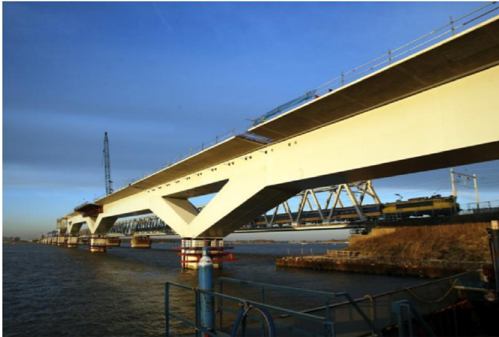
Figure 9: Bridge Hollands Diep
