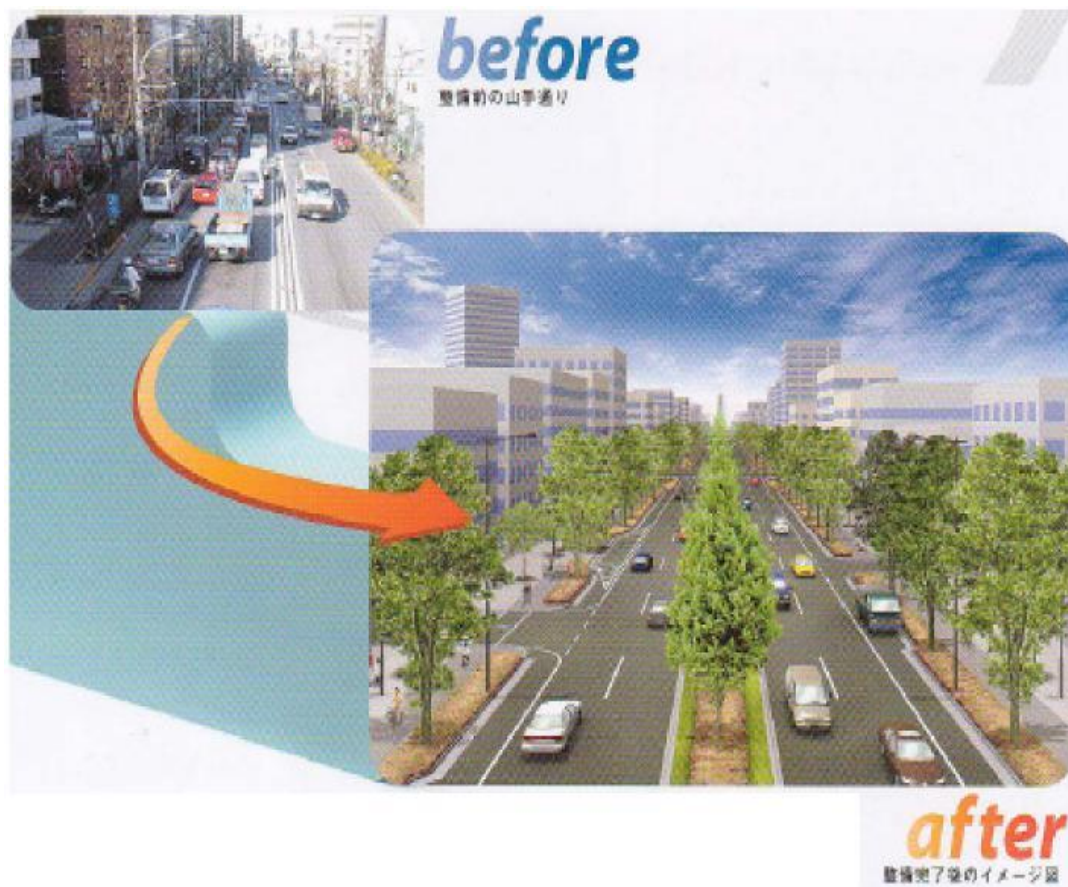
Figure 3: Upgrading of the 6th Circular Highway ('the Yamate Dori', 8.8km) from 22m to 40m width
