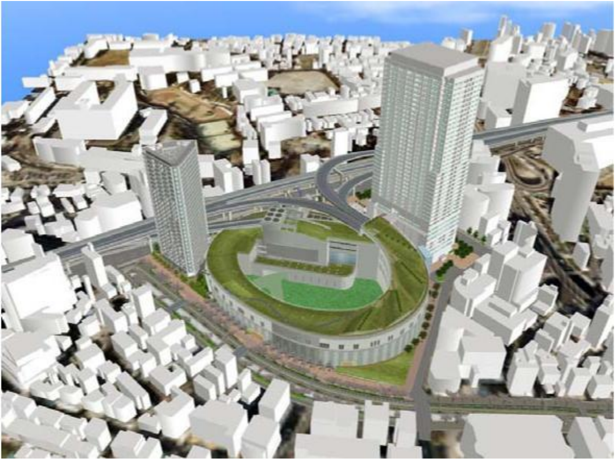
Figure 4: The Ohashi Urban Redevelopment Project - implemented with the project for the Ohashi junction building of the Metropolitan Expressway C2 Shinjuku Route (Nishishinjuku Junction – Ohashi Junction)
