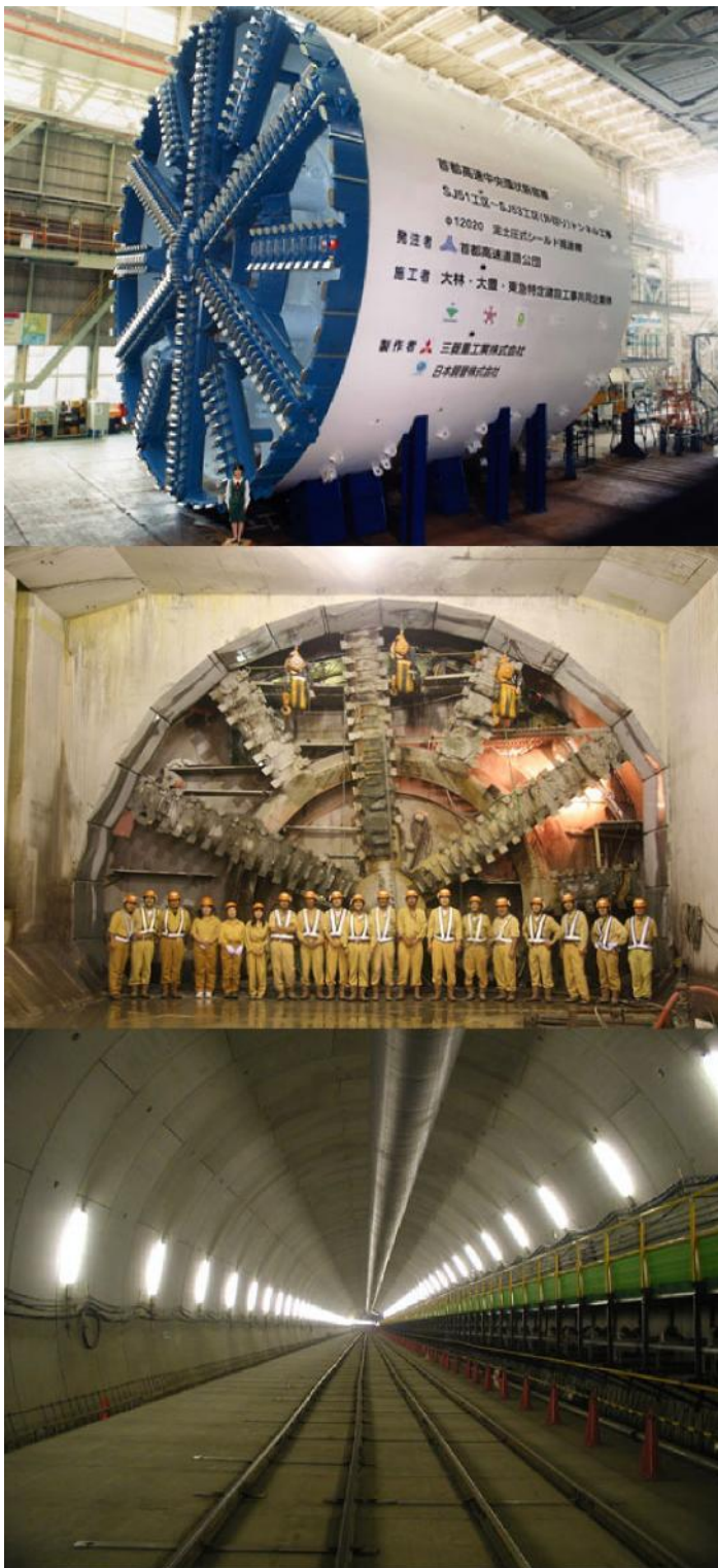
Figure 16: The earth pressure balance shield method
