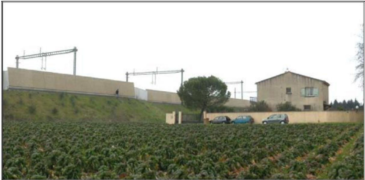
Figure 35: Noise-reduction screens on the TGV Med line
