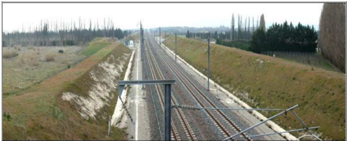
Figure 36: Merlon (natural noise-reduction screen) on the TGV Med line
