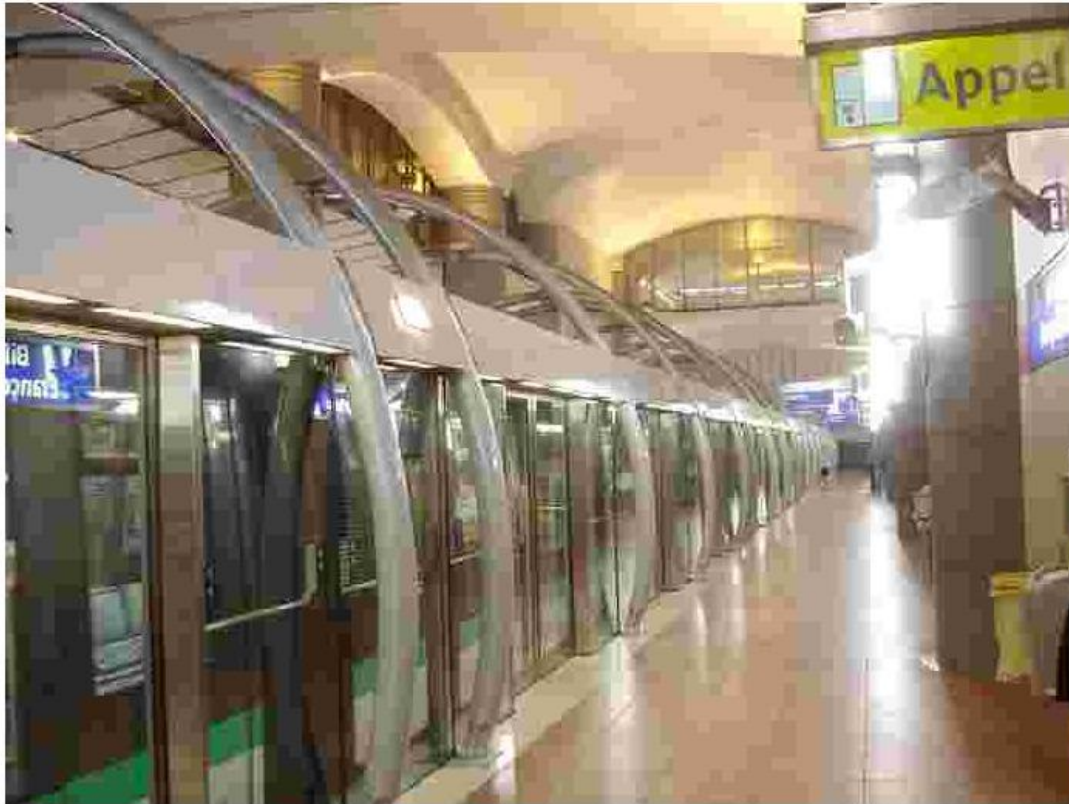
Figure 15: Platforms with glass doors (Bibliothèque F. Mitterrand station)
